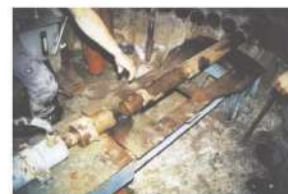
Fig. 16 Underexcavation at the Cathedral and the Sagrario
